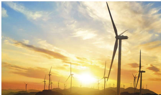
Aluminium Conductors Wind Power field
